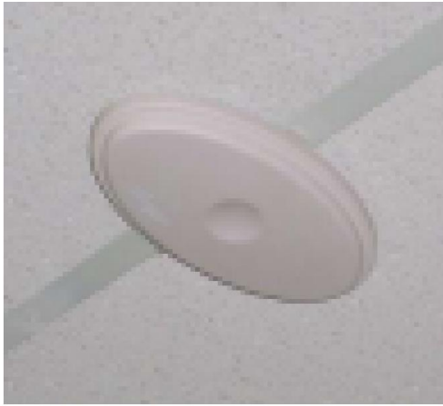
Installed Antenna
