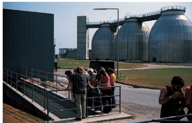
Figure 29.28 High-Efficiency Anaerobic Bioreactors Used for Sludge Digestion and Methane Production. These “egg-shaped” units are so well insulated that they maintain their temperature (39°C) without outside heating, and the methane can be burned to provide electricity. These reactors are located at Kiel, Germany.
