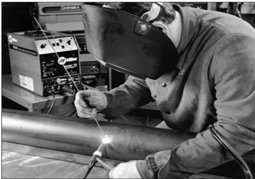
Figure 8.14 This welder (who happens to be left handed) demonstrates still another style of torch and filler rod manipulation used to accomplish a pipe weld.
