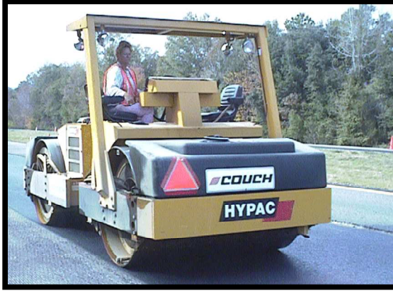
HMA Compaction
