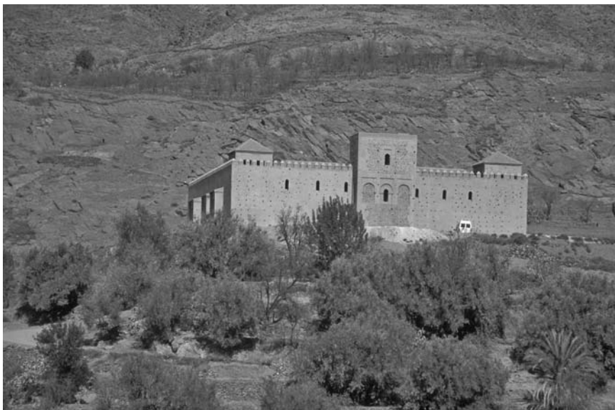
The Tinmal Mosque was part of the impregnable fortress in the High Atlas Mountains south of Marrakech, which served as the center of Almohad opposition to the Almoravids. (Photograph by the author.)
