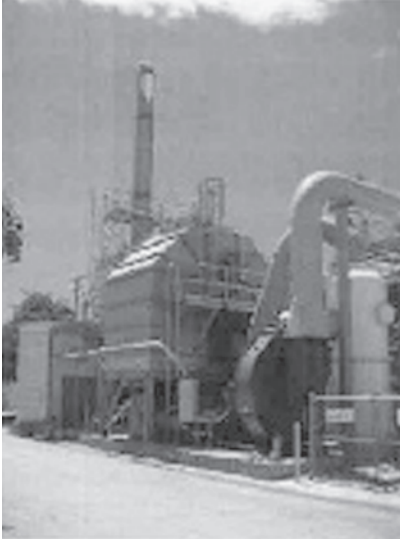
FIGURE 1 Thermal Oxidizer
