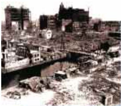
Left: The devastation of Tokyo in 1923 by a fire that broke out after an earthquake measuring 8.3 on the Richter scale.
